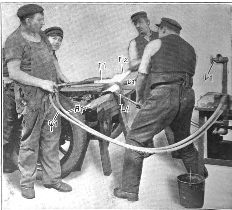
Fig. 2—Straightening bent dumb iron of frame by blast heating and using bending iron
